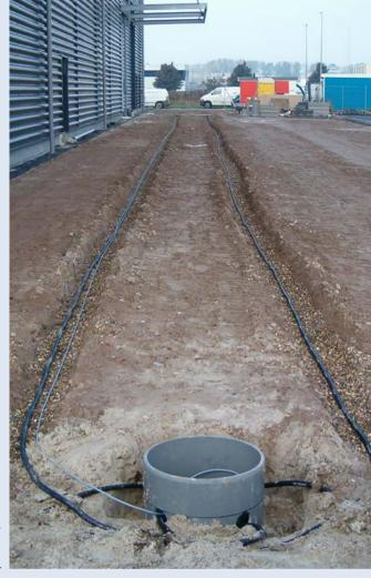
For ground detection, two cables (active system) or two tubes (passive system) are buried in the ground parallel to each other.
