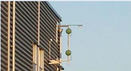
be provided to each corner of the roof. These add to the cost. What is also sometimes done is to place the sets with wall-mounting brackets on the upper part of the wall, just below the roof. Then you'll detect intruders as soon as they lean a ladder or other climbing equipment against the wall.
