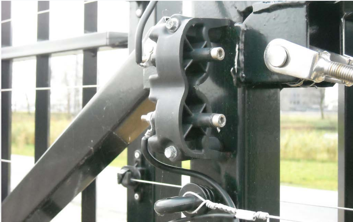
These contacts are used to transfer the voltage to the moving leaf of a swing or sliding gate
