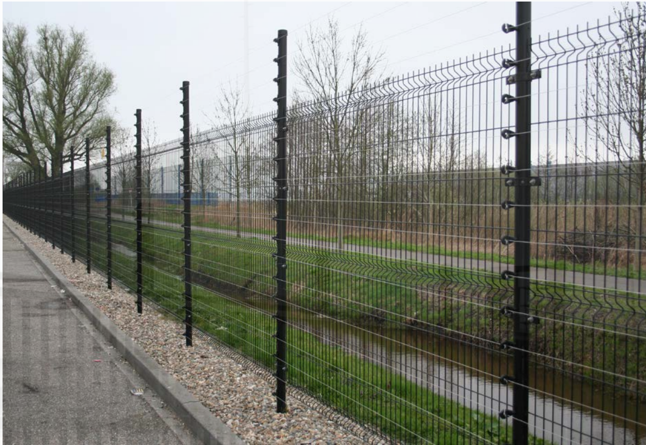
A strip of gravel with weed control fabric underneath ensures that no weeds grow along the power wires
