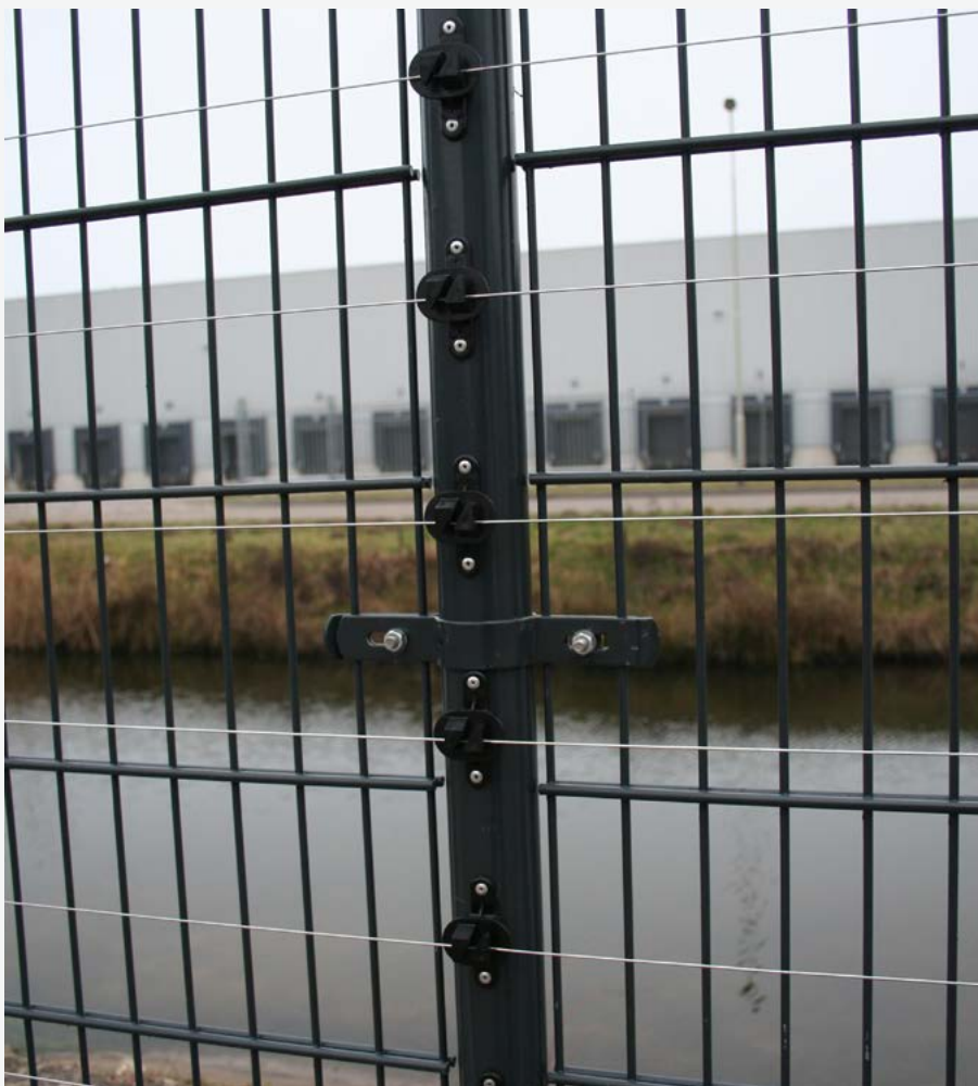
The wires of an electric fence are usually around 10 centimetres apart.
