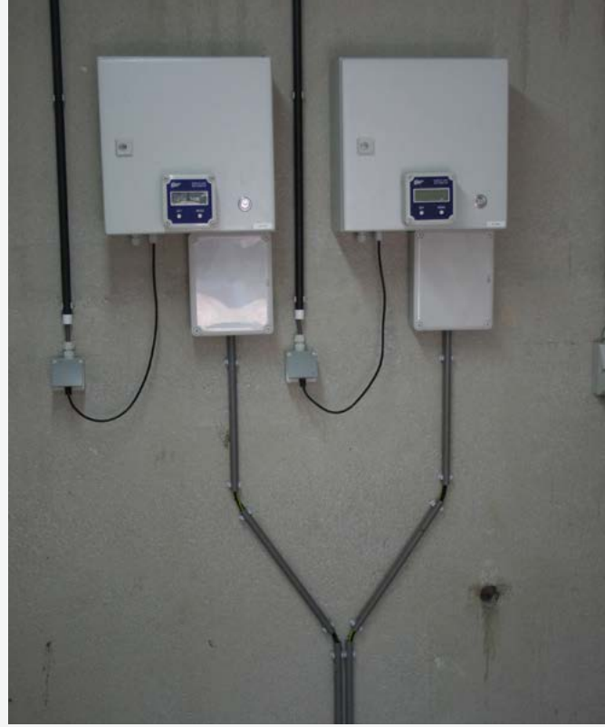
These switch boxes convert the 230-volt mains voltage to 7,000 or 8,000 volts.
