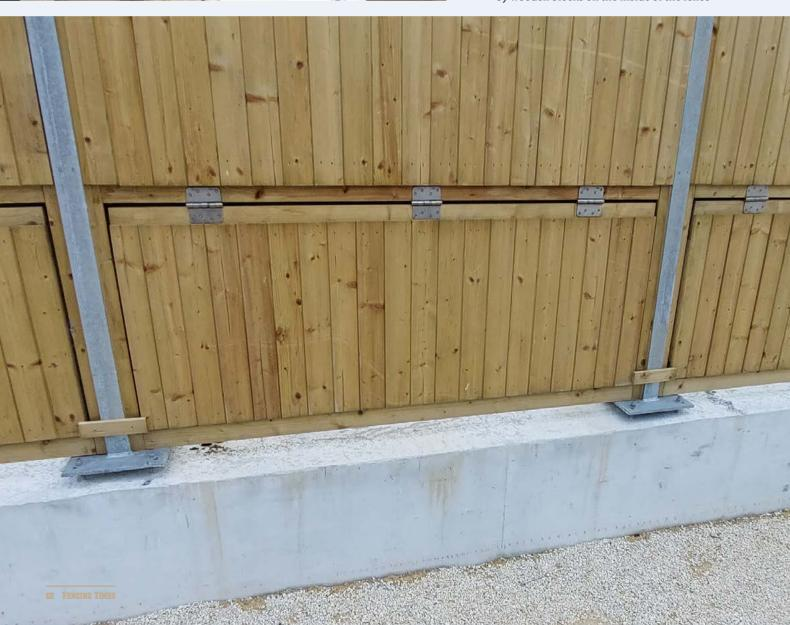
and these prevent the panel from flapping in the wind. If the water pressure becomes too great, the blocks break away. A wire panel that prevents the hinged panels from being pushed open from outside is fitted to the exterior, thus preserving perimeter security.
