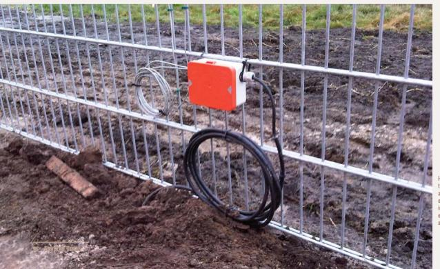
Here you can see the weld between the insensitive (black) cable and the sensitive (white) cable on the fence. Both cables are installed with a certain amount of excess length so there is enough available if repairs are required. the end of the sensor cable is a transition to a so-called single-mode cable, which returns the light to the analyser. This cable can simply be tie-wrapped to the fence here and there, but can also be buried in the ground. It has no detection capability.
