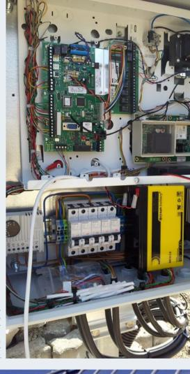
Field cabinet with power supply, emergency power supply, burglar alarm control panel with alerts via the mobile network, and a heater with a thermostat.
